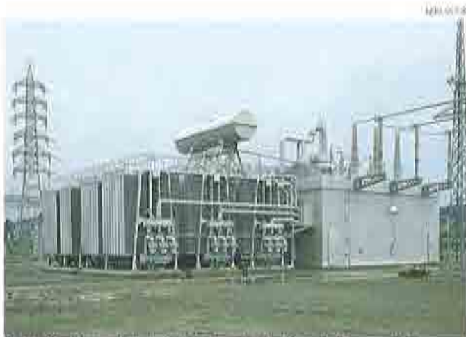
Photo 17 Separately installed forced-oil self-cooled type radiator
