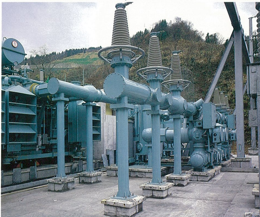
Photo 17 Transformer directly coupled to SF 6 gas insulated switchgear
