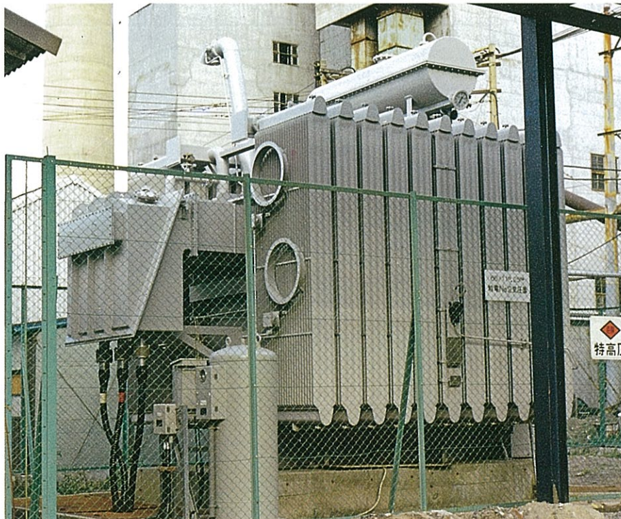
Photo 15 60kV oil-immersed elephant type transformer
