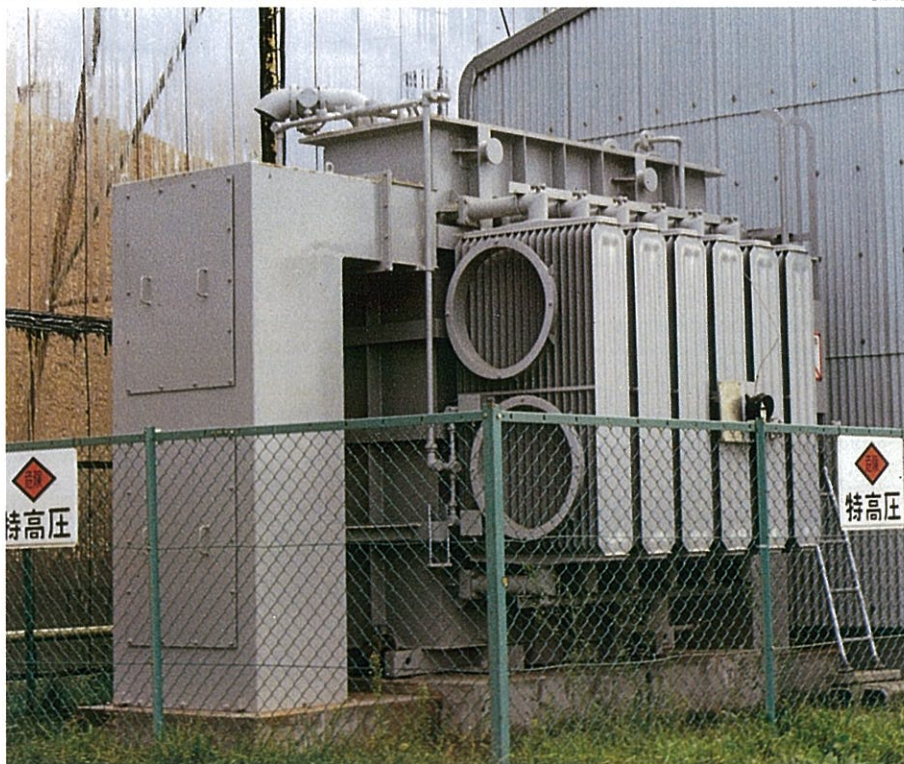
Photo 15 60kV oil-immersed elephant type transformer
