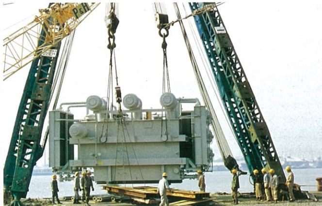
Photo 15 Transformer lifted with 350t gin pole crane
