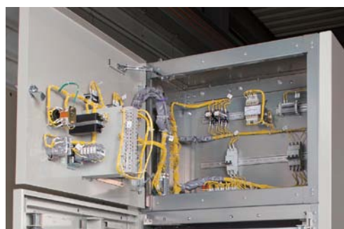
図3-8 制御室 Fig. 3-8 Control compartment
