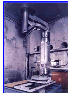
Fuel Handling Machine (Gripper)
