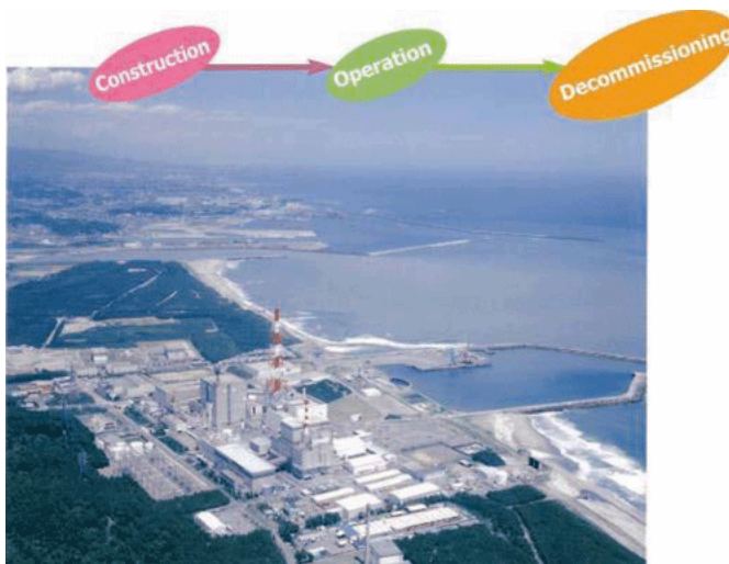
Full view of Tokai Power Station
