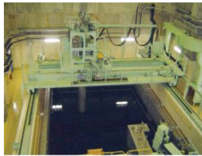
Spent Fuel Storage Facility
