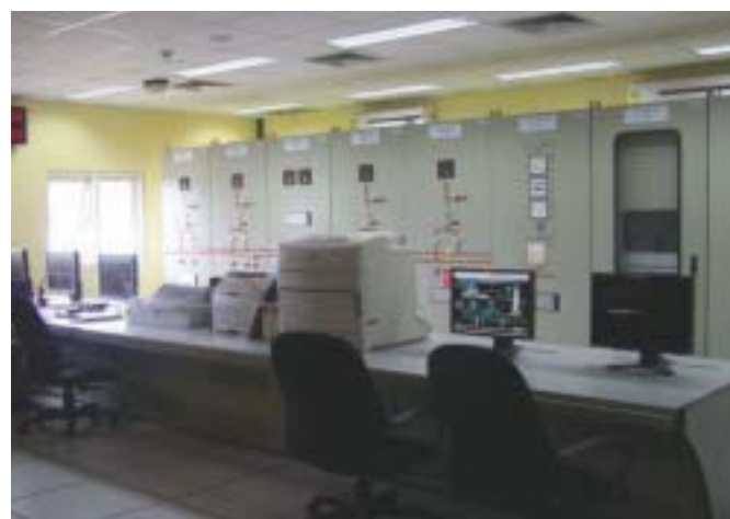
Central control room
