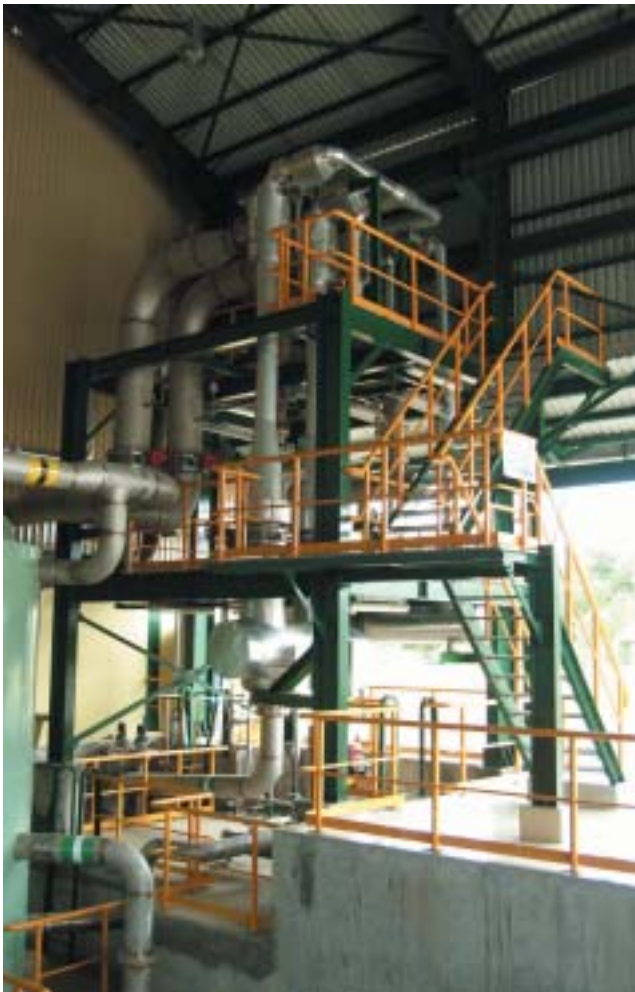
Gas removal system
