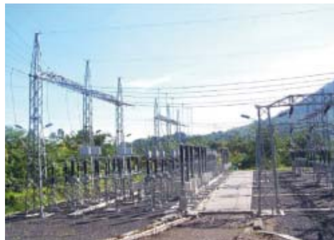
150kV system substation
