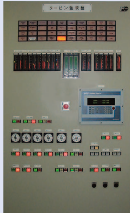
Turbine monitoring panel
