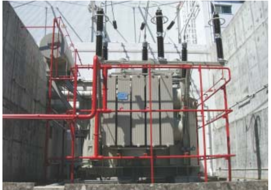
Generator transformer
