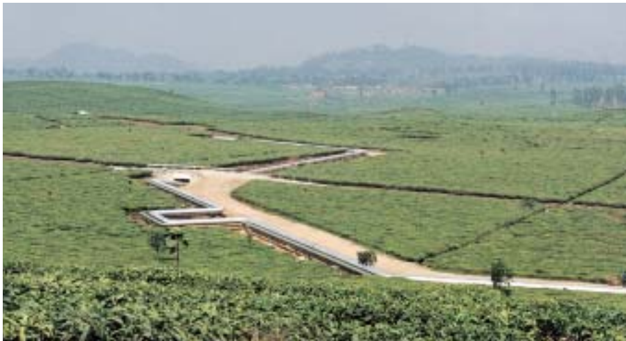
Pipeline from wellpad to separator station
