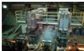
Steel rolling facilities
