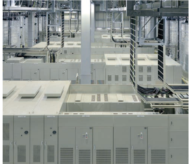
Minami-Hayakita Substation (Left: exterior view of the building Right: Fuji Electric power conditioning system inside the building)
