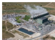
2010 A 140 MW geothermal power plant, the largest single-unit capacity in the world, started operation (The Nga Awa Purua Geothermal Power Station in New Zealand)
