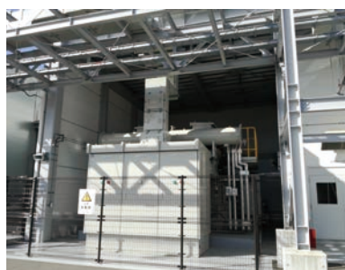
The S-Former Series delivered for the NEDO Development of Technologies for Realizing a Hydrogen Society (For 10 MW class large-scale water-electrolyzing apparatus system)
