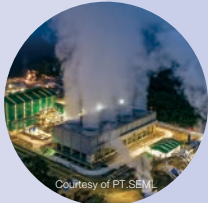
Geothermal power generation
