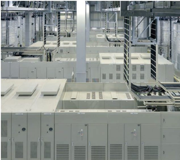
Minami-Hayakita Substation (Left: exterior view of the building Right: Fuji Electric power conditioning system inside the building)
