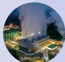
Geothermal power generation
