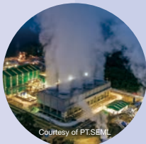
Geothermal power generation
