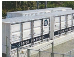
Power storage systems
