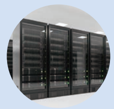
Power supply and facility systems
