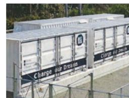
Power storage systems
