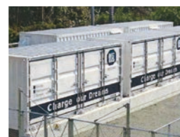
Power storage systems
