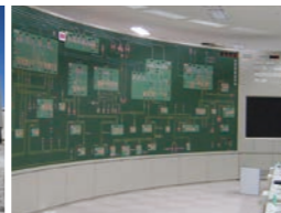
Monitoring and control systems for power grids
