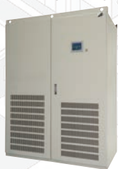
Uninterruptible power system (UPS)
