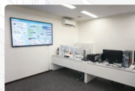
In the control building at the Soma IHI Green Energy Center (energy management system)
