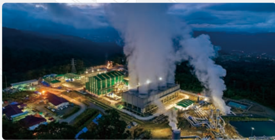
Muara Laboh Geothermal Power Plant (Courtesy of PT. SEML)
