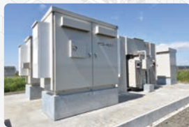
Power conditioning system
