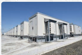
Storage battery facilities
