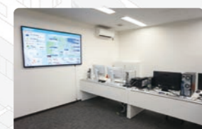
In the control building at the Soma IHI Green Energy Center (energy management system)
