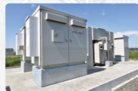
Power conditioning system
