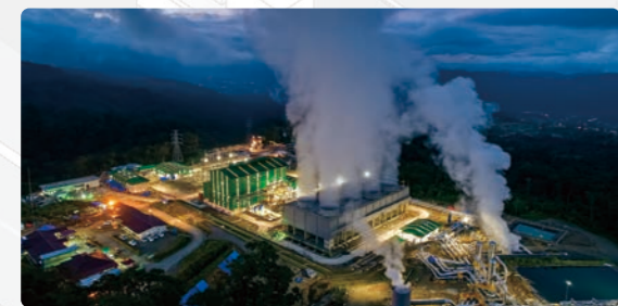
Muara Laboh Geothermal Power Plant (Courtesy of PT. SEML)
