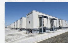
Storage battery facilities
