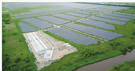
Suzuran Kushiro-cho Solar Power Plant (Hokkaido, Japan)
