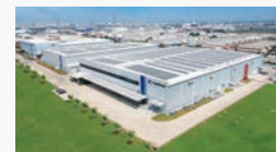
Fuji Electric Manufacturing (Thailand) Co., Ltd.
