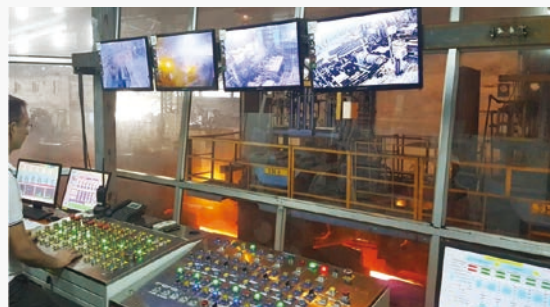
Monitoring and control room (steel plant in India)
