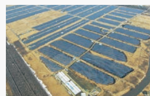
Suzuran Kushiro-cho Solar Power Plant (Hokkaido, Japan)
