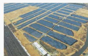
Suzuran Kushiro-cho Solar Power Plant (Hokkaido, Japan)
