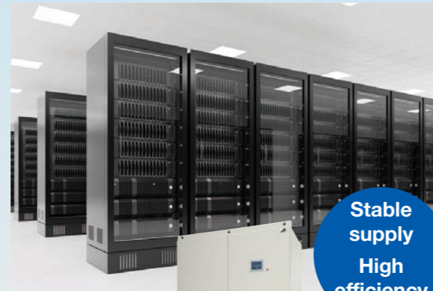
All-inclusive provision of highly reliable and highly efficient electric equipment for data centers, from system design through to installation and maintenance services
