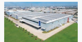
Fuji Electric Manufacturing (Thailand) Co., Ltd.
