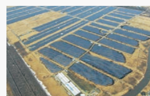
Suzuran Kushiro-cho Solar Power Plant (Hokkaido, Japan)
