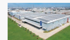
Fuji Electric Manufacturing (Thailand) Co., Ltd.
