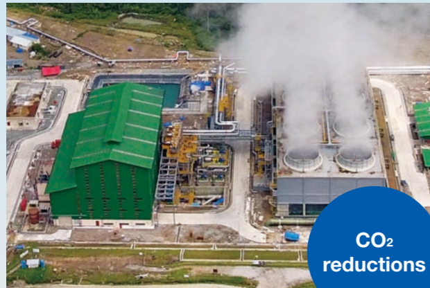
Muara Laboh Geothermal Power Plant in Indonesia Power generation capacity equivalent to the power usage of 420,000 households on the Indonesian island of Sumatra (Source: Sumitomo Corporation website)
