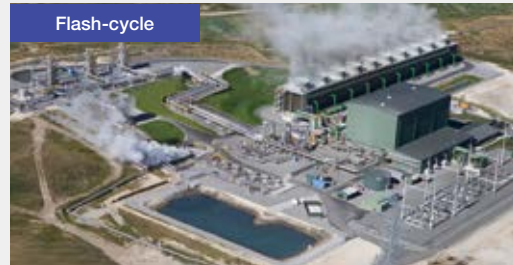
Nga Awa Purua Geothermal Power Station (140 MW generation capacity, New Zealand)
