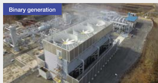
Takigami Binary Geothermal Power Station of Idemitsu Oita Geothermal Co., Ltd. (5.05 MW generation capacity, Oita Prefecture, Japan)
