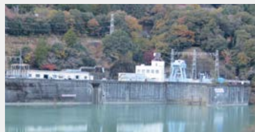
Akiha No. 1 Power Station of Electric Power Development Co., Ltd. (47.2 MW, Shizuoka Prefecture, Japan)
