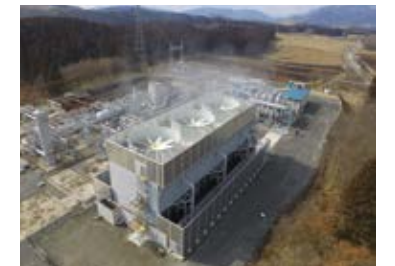
Takigami Binary Geothermal Power Station
