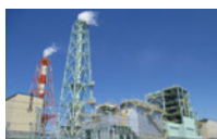
Nagoya Power Plant 2 (Biomass)
