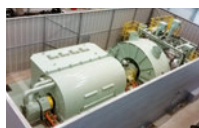
Steam turbine and generator
