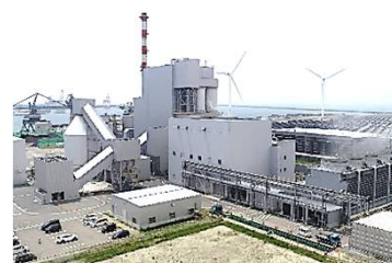
Biomass power plant
