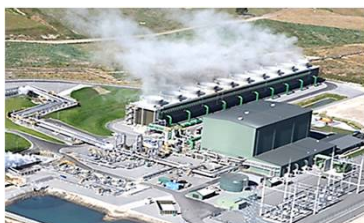
Geothermal power plant (flash)
