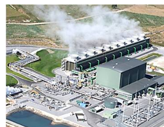
Geothermal power plant (flash)
