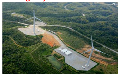
Ogimi wind power plant verification research facilities (4,500 kWh lead-acid storage battery)
