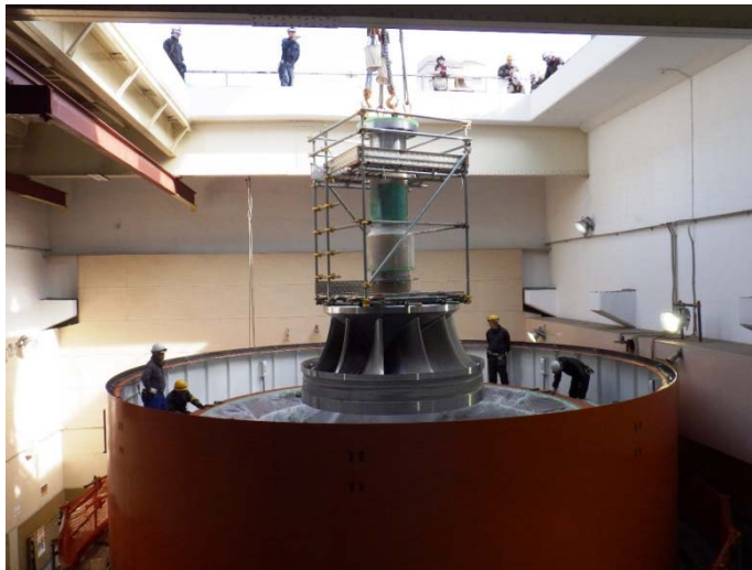
【Turbine and Generator Upgrades】
