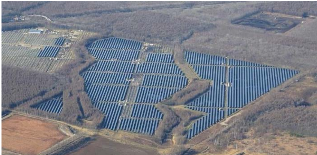
Tomakomai Mega Solar Power Station No. 1 of GPD Sakura Solar (EPC project with generation capacity of 38 MW of DC power and 25 MW of AC power)
