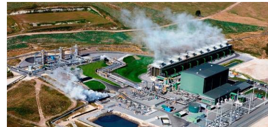
Nga Awa Purua Geothermal Power Plant (New Zealand)
