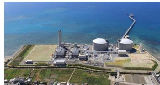
Okinawa Electric Power Company Yoshinoura Thermal Power Station (Japan)
