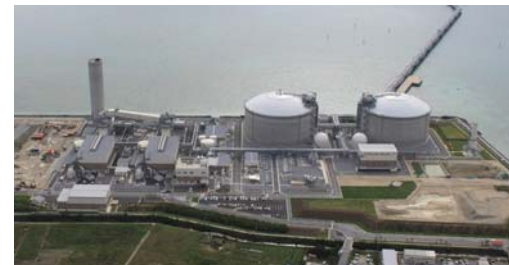
Yoshinoura Thermal Power Station
