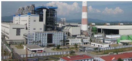
Haiphong Coal-Fired Thermal Power Station in Vietnam
