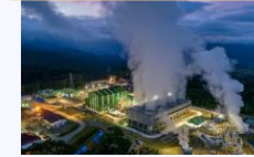
Geothermal power generation plants
