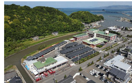
Solar power generation system for powering Akune City (Photograph provided by Trust Bank Akune)
