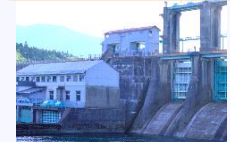
Hydropower generation plants
