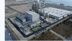
Biomass power generation plants
