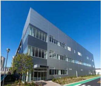
Plant system building
