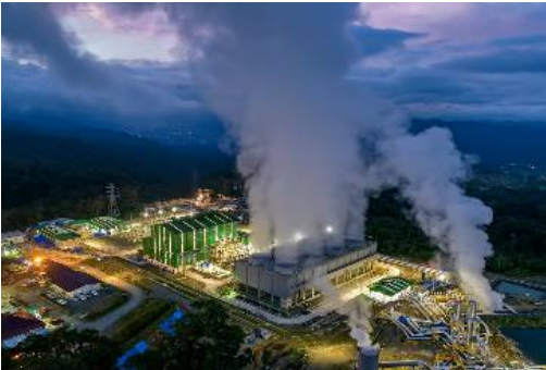
Muara Laboh Geothermal Power Plant (Photograph provided by PT. Supreme Energy Muara Laboh)
