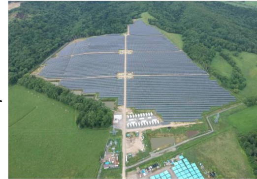
GPD Oboro Solar Power Plant (Photograph provided by Green Power Development Corporation of Japan)
