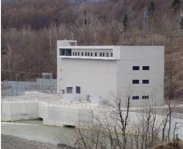
Shimizu Sawa Hydro Power Plant (Photograph provided by Hokkaido Prefectural Enterprise Bureau)
