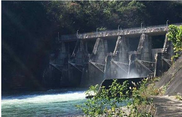
Sasadaira Power Station (Photograph provided by TEPCO Renewable Power, Inc.)
