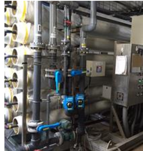
Wastewater recovery system
