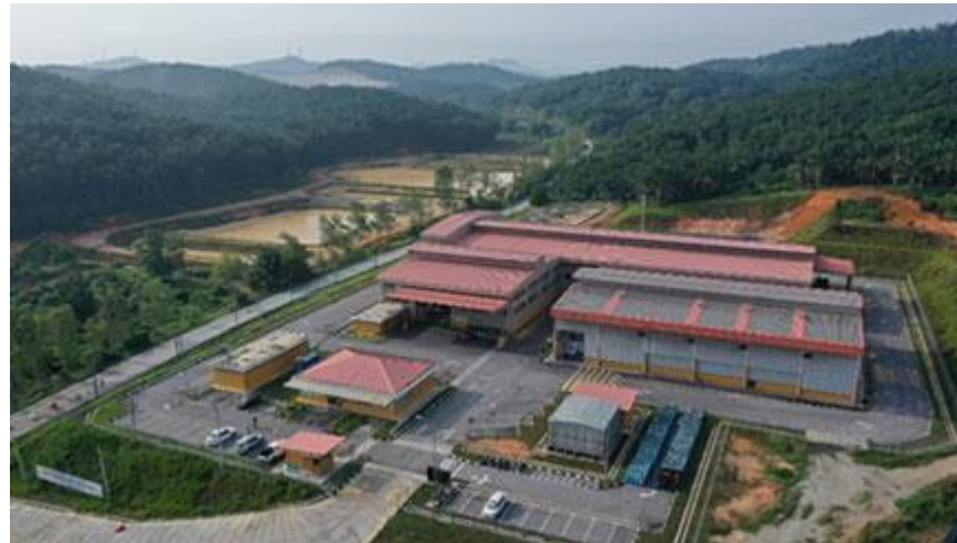
AKBK Sustainable Resource Management Centre waste recycling plant
