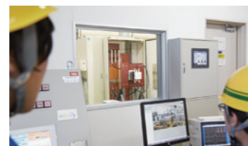
Breaking test to verify safety during large current flow accidents
