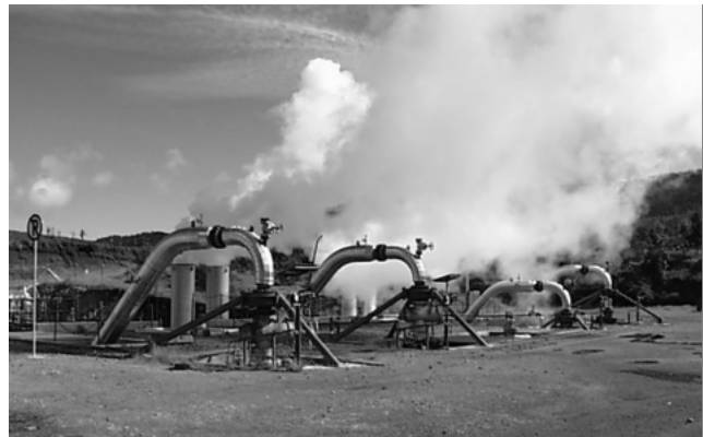
Fig.8 Production wellpad (WWQ)
