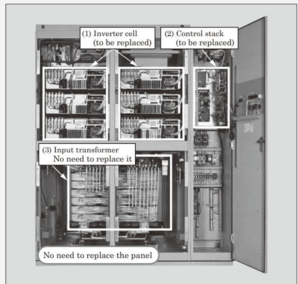
Fig.8 Image of medium-voltage inverter retrofit
