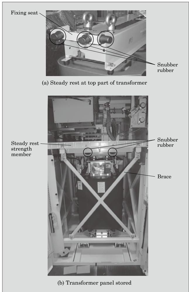
Fig.7 Steady-rest structure at top part of transformer
