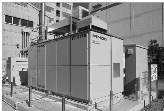
Fig.1 Phosphoric acid fuel cell “FP-100i”
