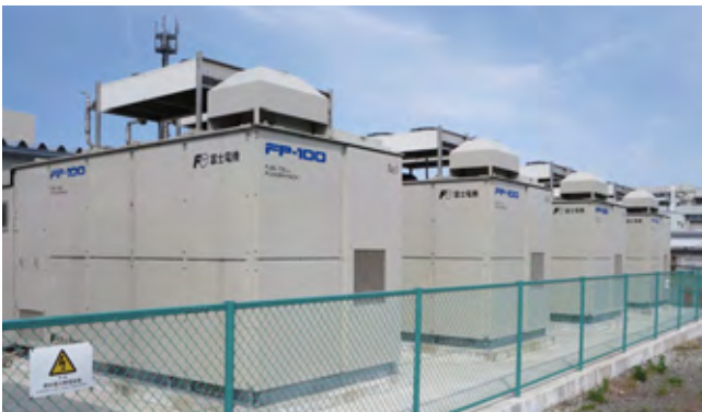
Fuel cells installed at a model factory (Yamanashi Factory) under Fuji Electric's Smart Factory Initiative
