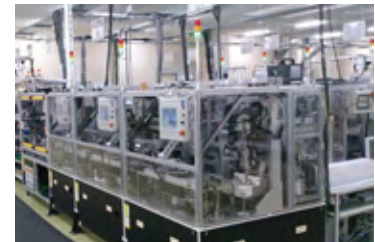
An automated inverter assembly line (Suzuka Factory)
