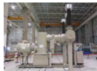
Gas-insulated switchgear
