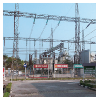
Industrial park substation
