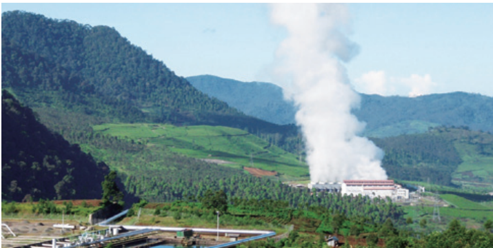
Wayang Windu Geothermal Power Station (Indonesia)
