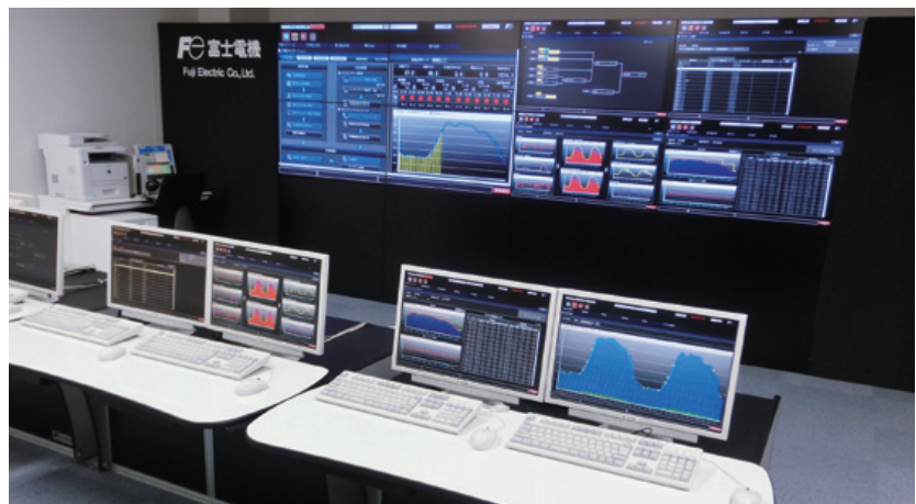
Cluster Energy Management System (CEMS)
