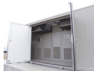
Power conditioners in an outdoor container at the Moji Power Plant
