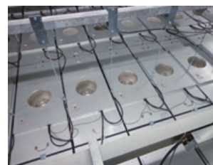
The Fuji Electric Fan Filter Unit with Inverter (clean room upper chamber) controls airflow optimally for each work area
