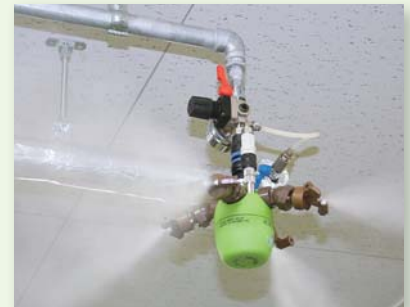
Humidity-adjusting dry fog
