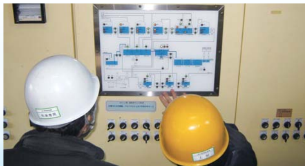
On-site inspection of Green Factory / Green Office evaluation at Kawasaki Factory
