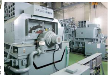
Cogeneration System Unit 3
