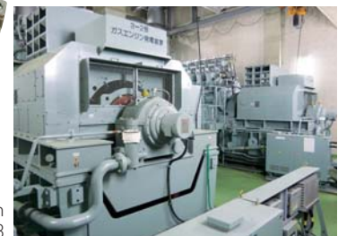
Cogeneration System Unit 3
