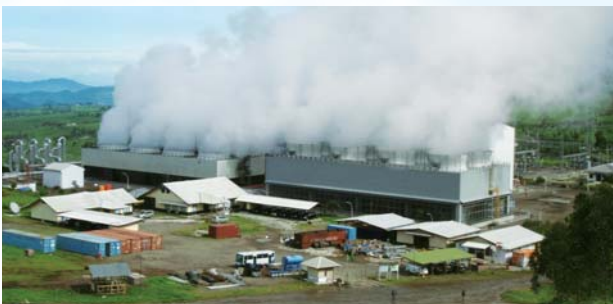
Wayang Windu Geothermal Power Station in Indonesia
