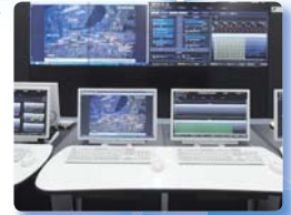
Community energy management system
