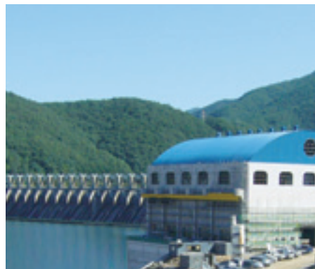
Hydraulic power plant (South Korea)
