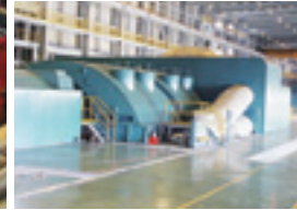
Thermal power generation facilities
