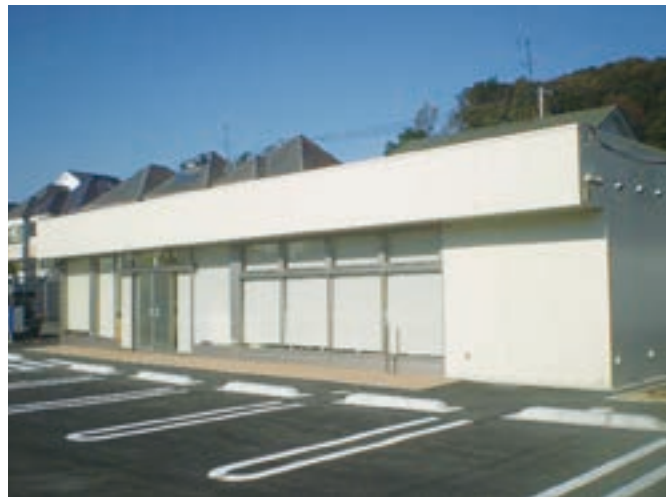
Environmentally friendly store (Ecolo panels)
