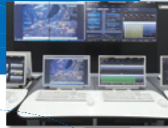
Cluster Energy Management System
