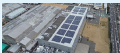
Solar power generation equipment at Suzuka Factory
